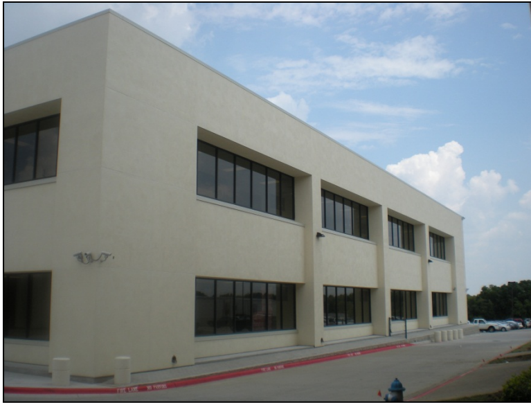
Exterior view of new Science Addition 9/15/10
