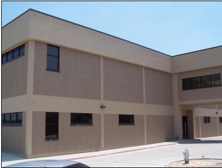
View of Bldg. B Addition
