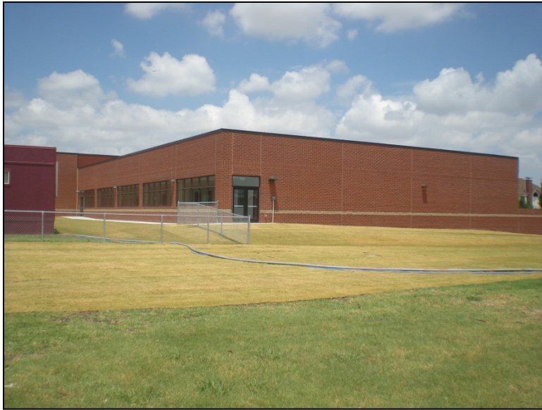
View of Classroom/Kitchen Addition 6/18/10
