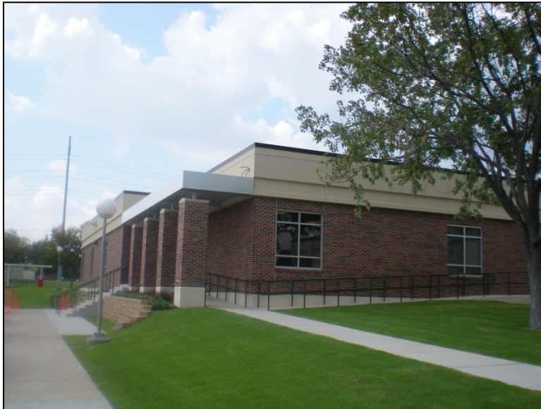
View of new Classroom Addition
