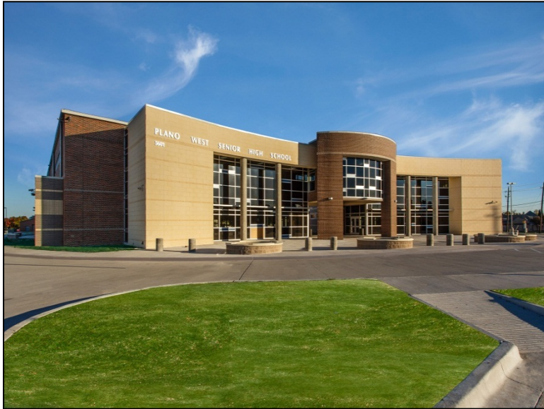
View of new CTE & Art Building
